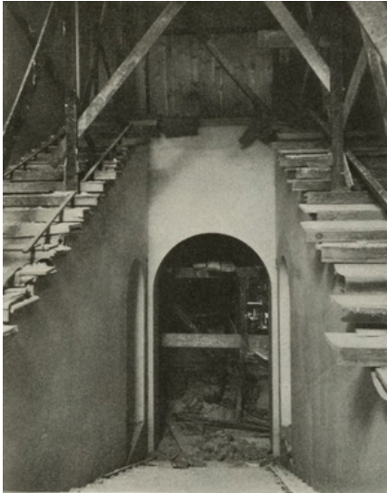
The principal White House stairway during the renovation process, 1902.
